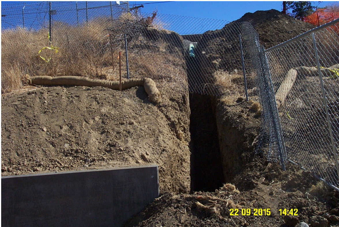
Figure 3 – Installation of new storm drain pipe and trench off of Putah Creek Road.
