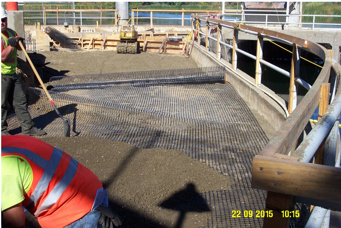
Figure 2 – Installation of Geogrid fabric and aggregate base.
