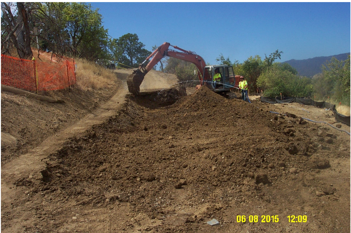
Figure 4 – Excavation of entire roadway fill for the West Side Access Road.
