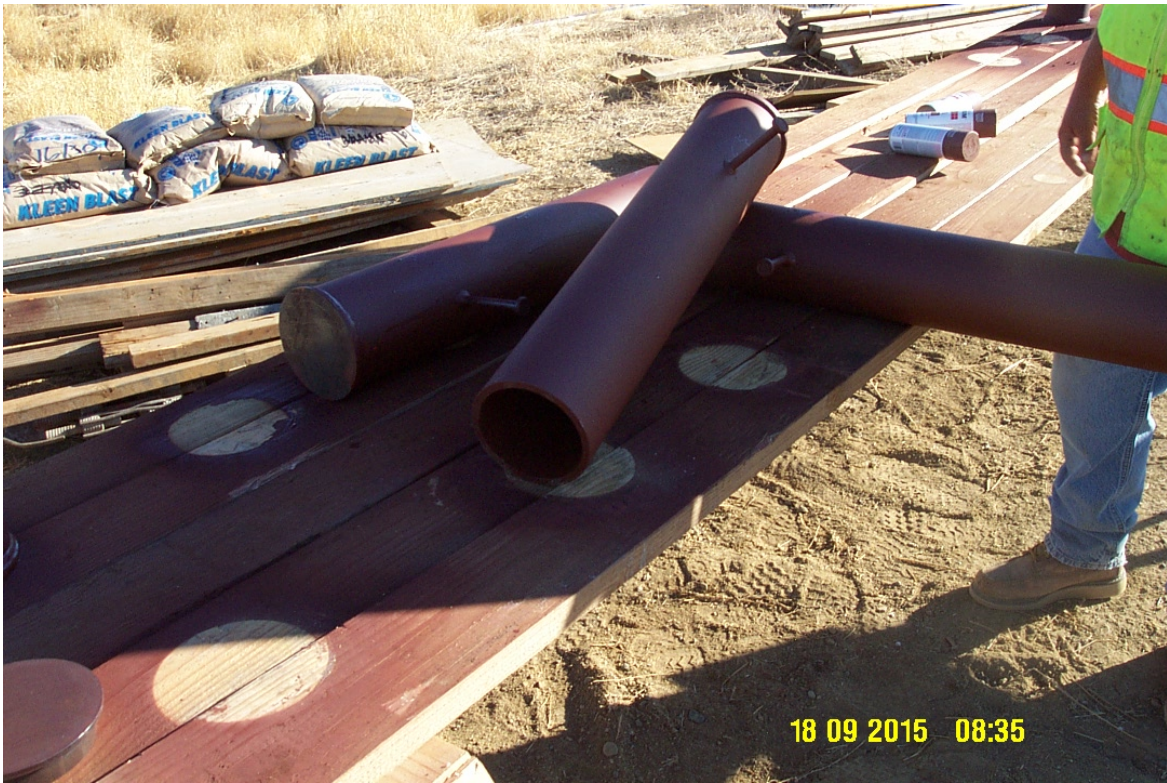
Figure 1 – Priming the steel bollards (guard posts) to prevent rust
