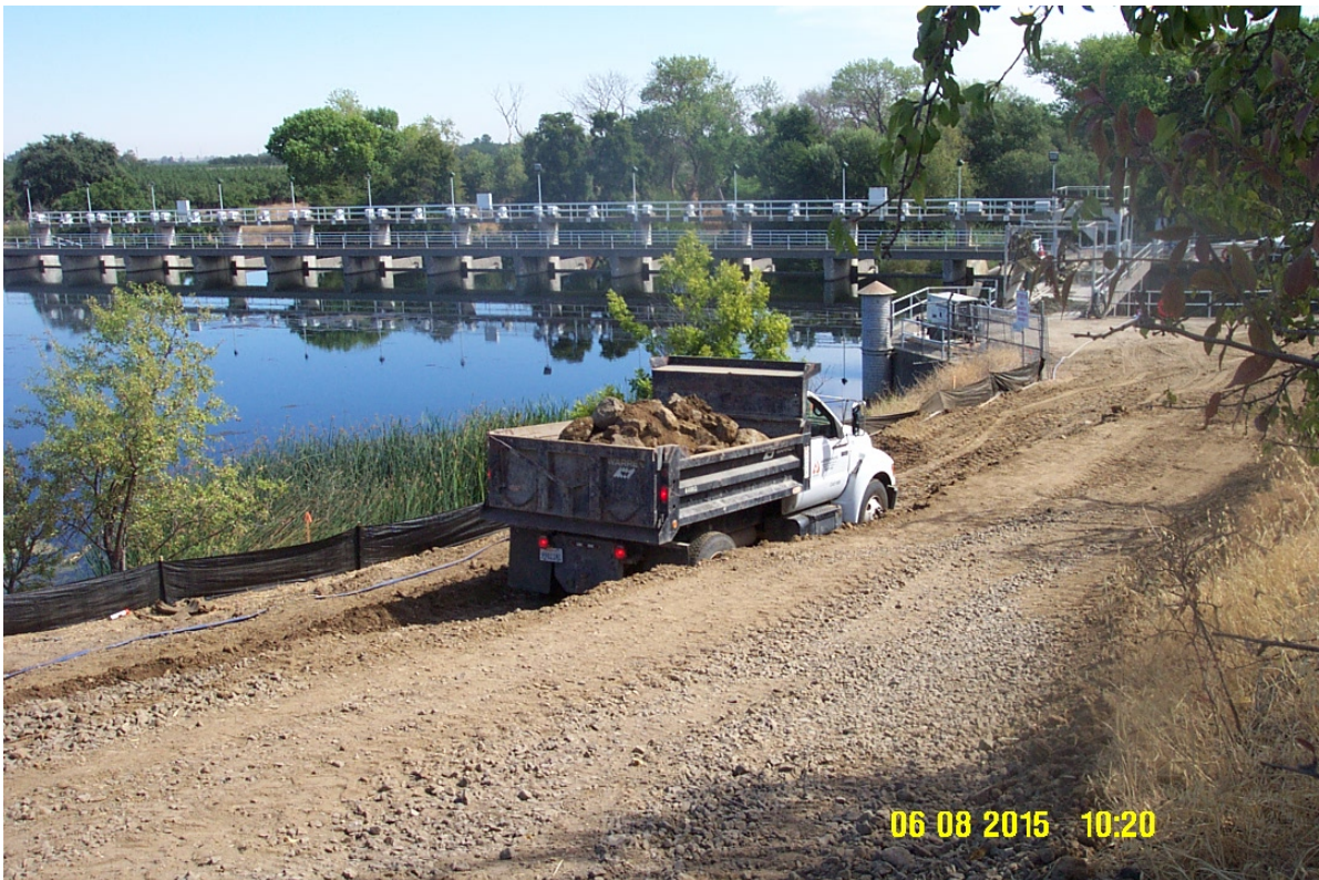
Figure 6 – Hauling away of large engineering rock from the old fill material.
