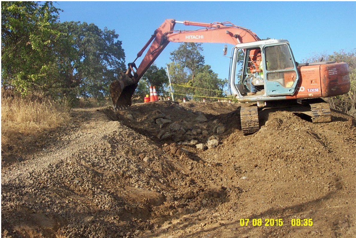
Figure 5 – Excavation of roadway with large engineering rock in the old fill material.
